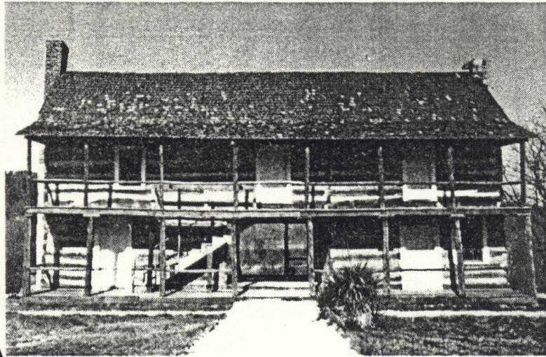
The Wolf House is the most historical building in Baxter County.
