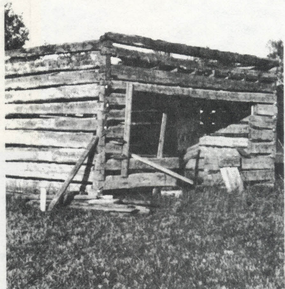
The Log Cabin's logs are all in place, awaiting the roof.
