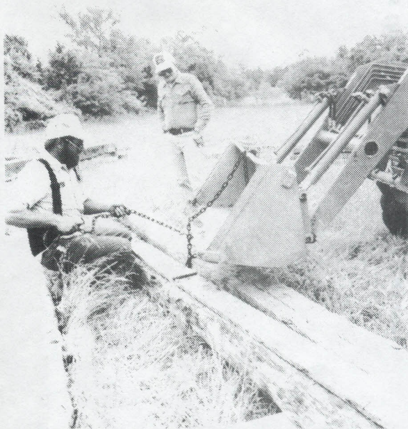
Talbert/Leonard Cabin logs being sorted for installation in Cooper Park
